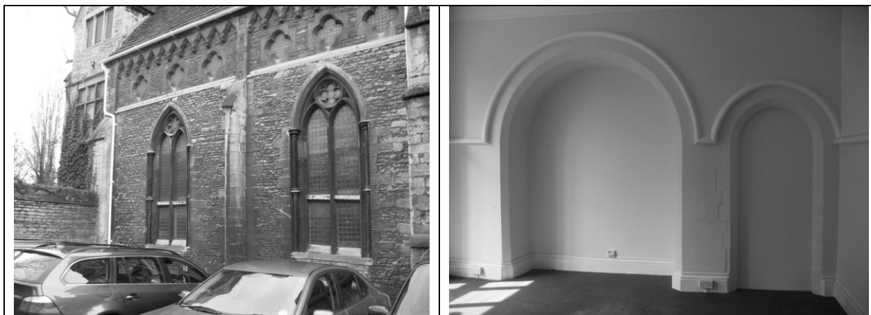
The north elevation of Archdeaconry House (left), and the blocked arches/doors in the western ground floor room (right).
