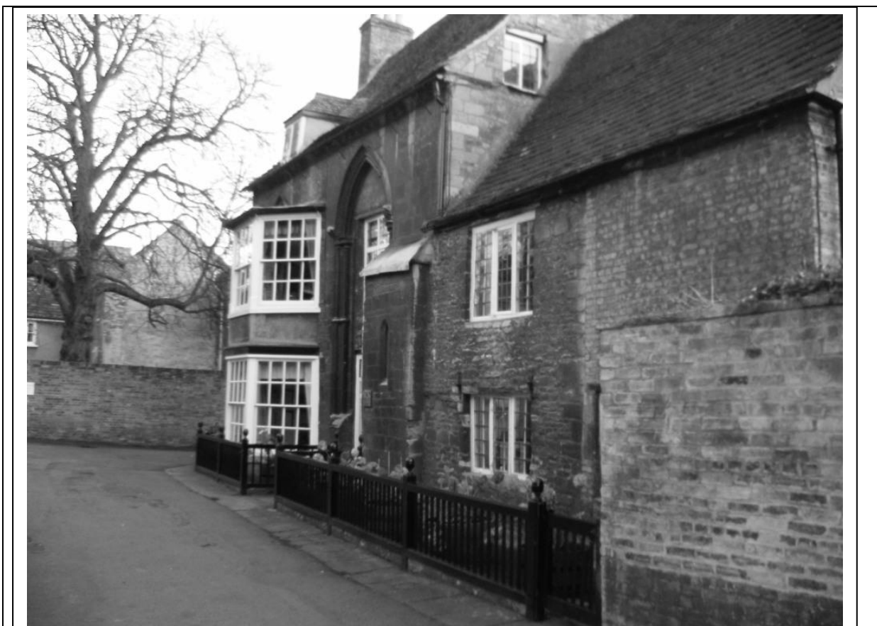
The north elevation of 19 Minster Precincts.
