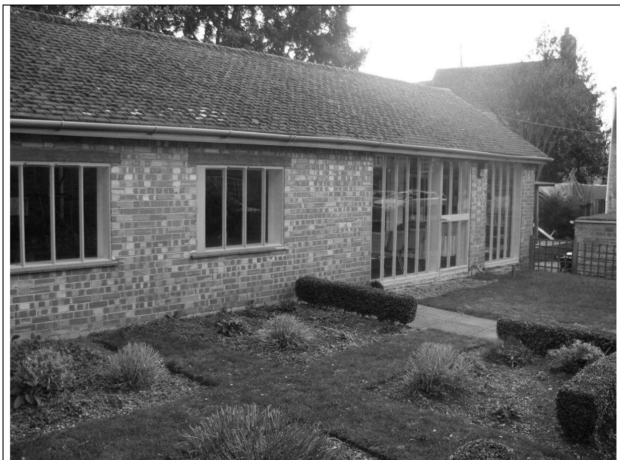
The education centre and herb garden, seen from the north-west.
