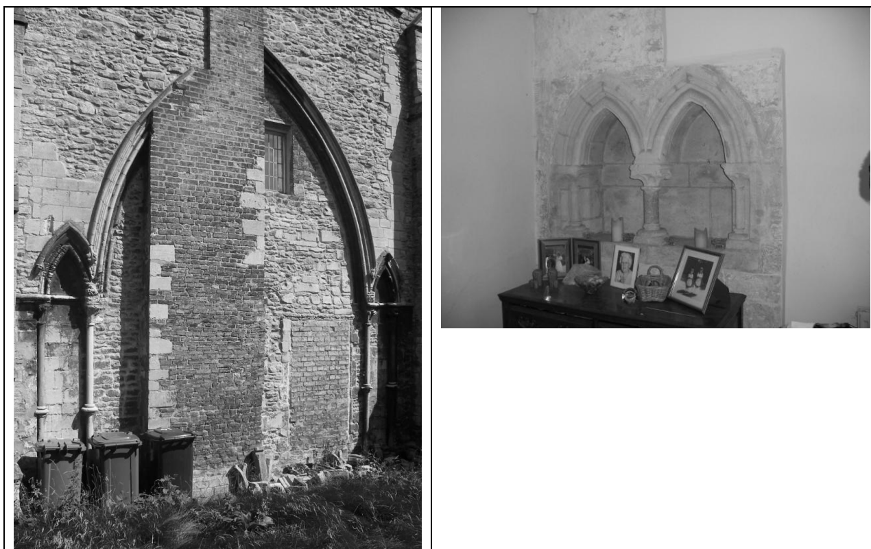
The blocked chancel arch in the east elevation of the Precentor's Lodging (left), and the piscina (right).
