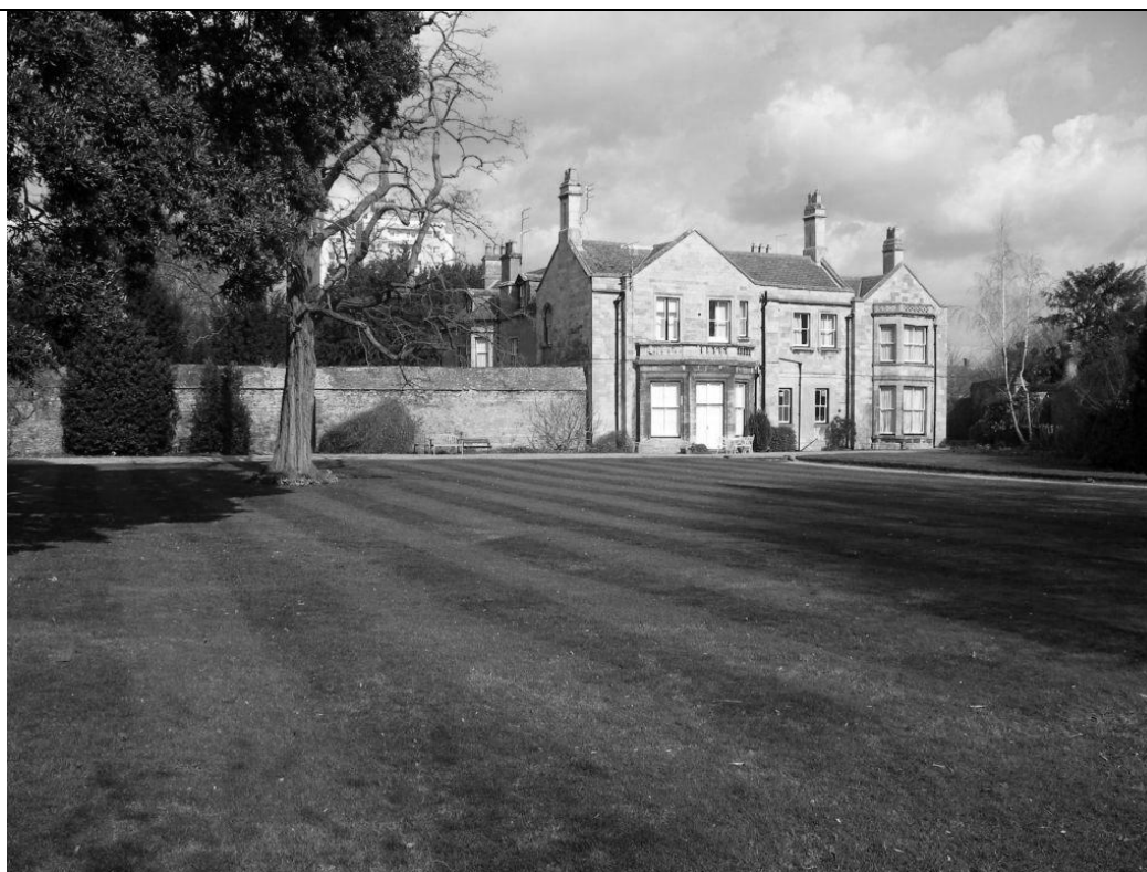
The west elevation of the Vineyard.
