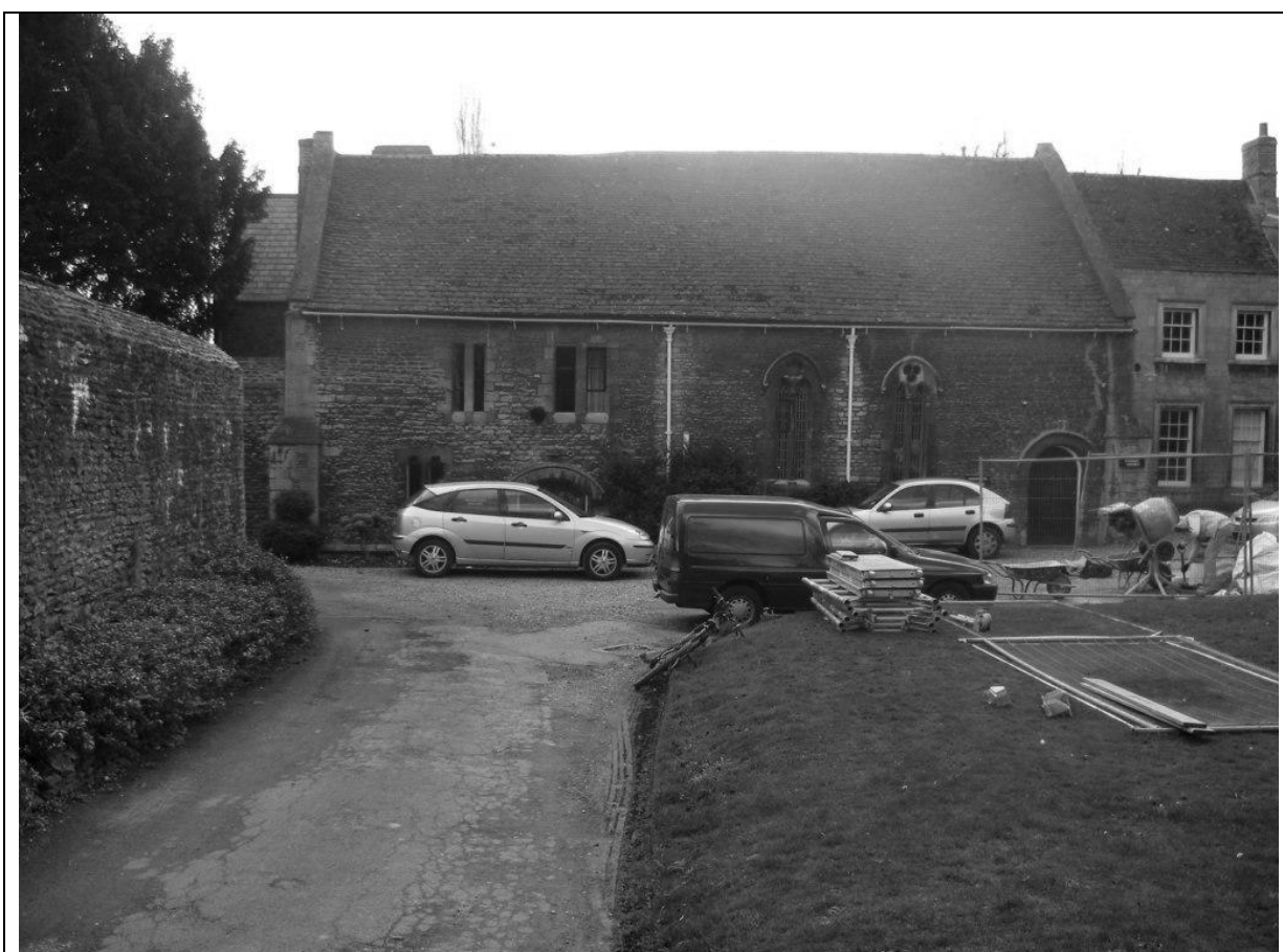
Canonry House (central part with lancet windows, and right with sashes) and the Precentor's Lodging (left) with mullioned windows. The left-hand of the two downspouts marks the approximate boundary between the two residences.
