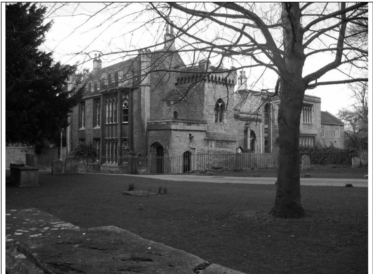
Little Prior's Gate – the south (left) and east (right) elevations, with the Deanery further to the right.
