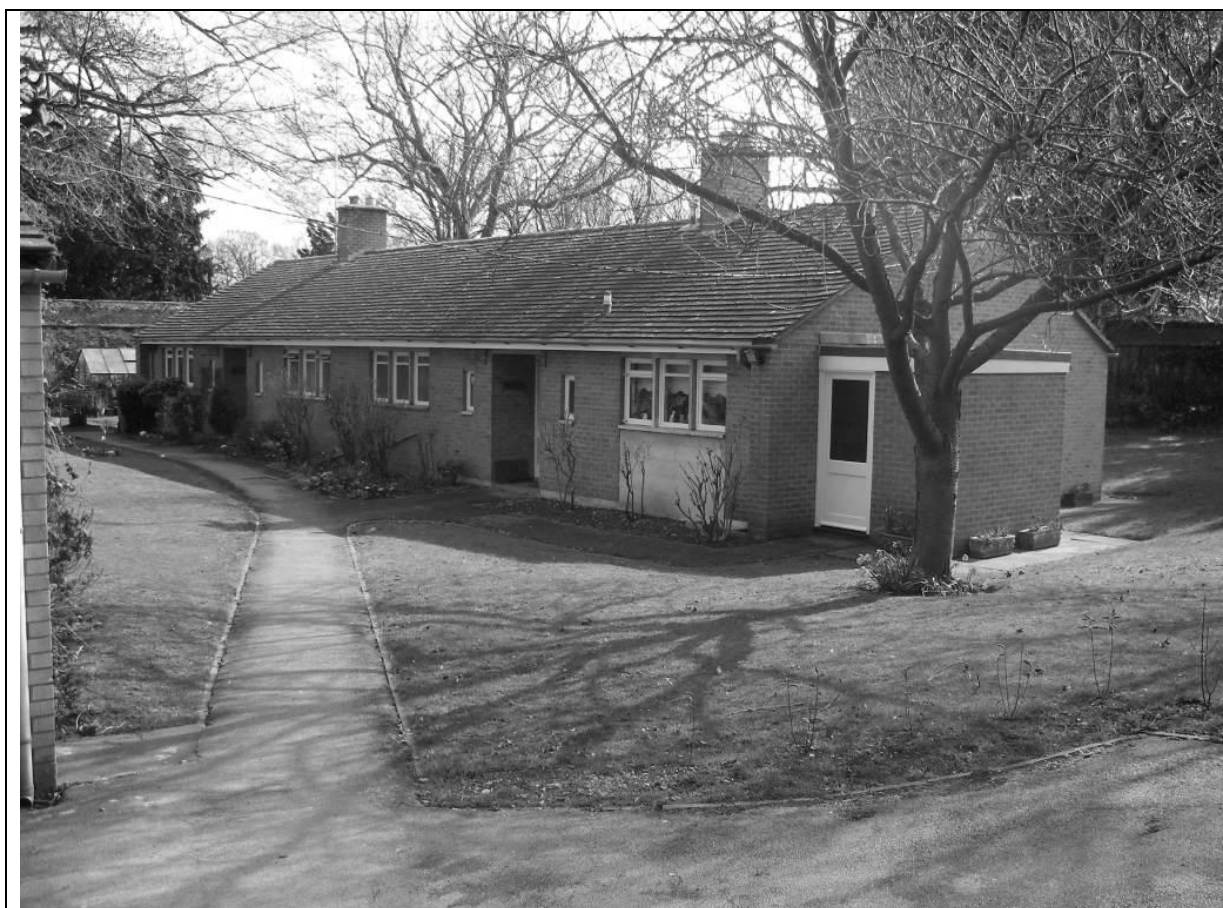
The north elevation of Ashton House and Mandell House.
