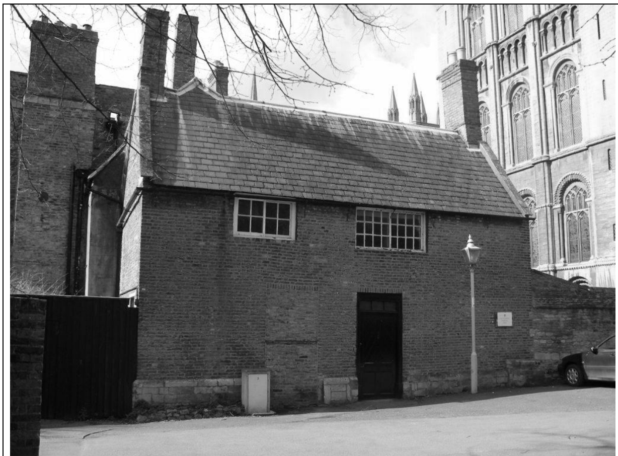
Laurel Court Cottage – east elevation.
