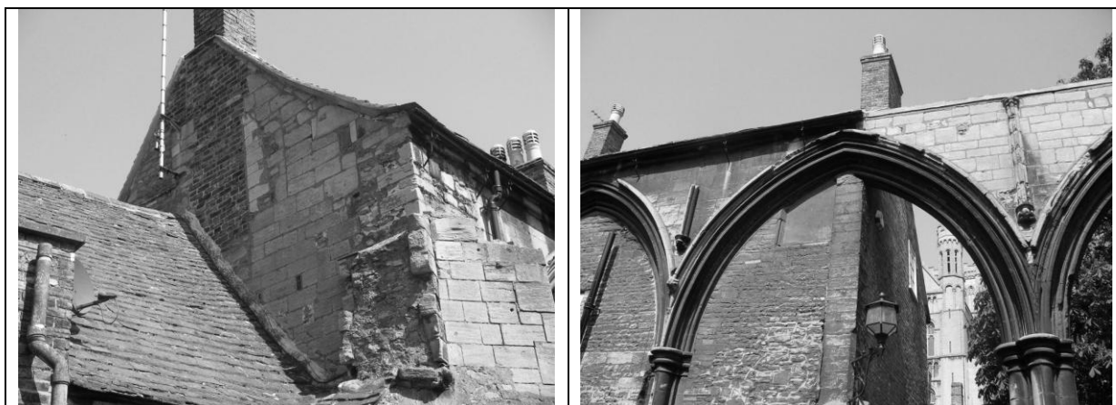
19 Minster Precincts: the west gable of the Infirmary Hall with the later extension to it (left), and walls of the house inserted into the Hall arcading (right).
